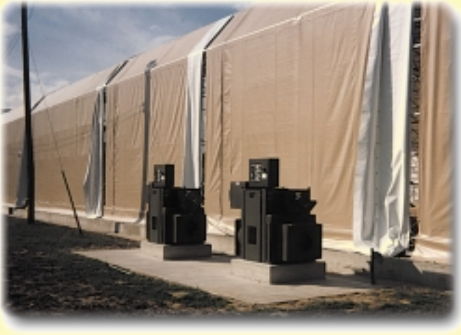
Dry The Whole Building
